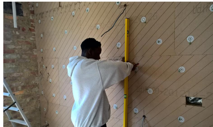
Installation of wood fibre insulation boards internally (© Back to Earth & ASBP)
