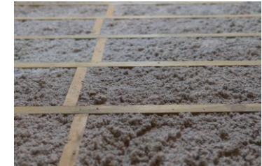
Cellulose- made from recycled paper
