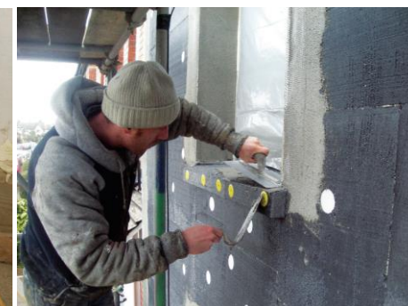
Photo of window install in Enerphit retrofit (© Passivehouseplus)
