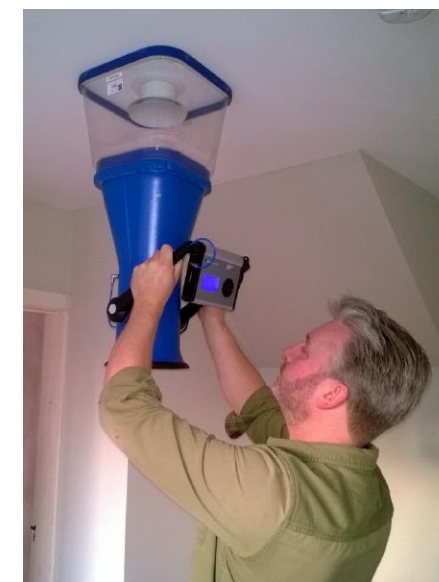
Flow rate measurement: image of MVHR system being commissioned (© Fourwalls)
